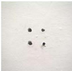
2) Drill four holes (6 millimeter in diameter) and insert wall plugs / screw anchors.
