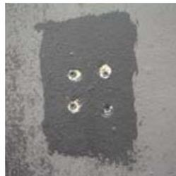
3) Apply two coats of shielding paint to area where the ground connection plate will be mounted. Allow ample time to dry.
