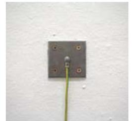
7) Connect cable to ground securely. E.g. use enclosed clip to connect cable to blank / bare heating pipe, or connect to grounding bar in fuse box.
